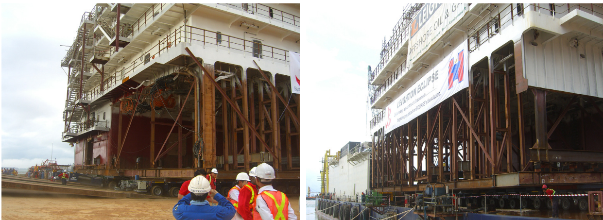
Pictures: Load out of Leighton Eclipse's accommodation and pipe laying barge
