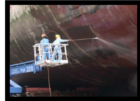
High Pressure Wash
